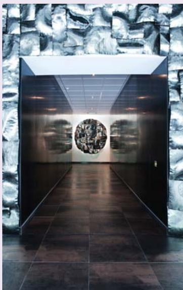
hand in hand at Montanstahl, Stumm says. The wall cladding in the entrance hall of the building also makes wide use of stainless, consisting of 1.4301 (304). The three unique sculptures in front of the building, commissioned for the site, are fabricated from 1.4404. Hailed among the frontline contemporary artists of the day, artist Xhixha has a special relationship with stainless steel, which is his primary raw material in sculptures.
